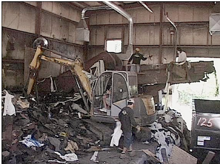
Picture 13 - Grapple Crane Servicing Indoor Loads of Mixed Roofing Materials (Together with Floor Picker Coupled With Elevated Sort Line)
