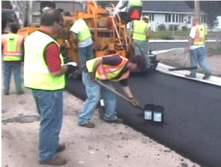
Picture 19 - HMA Sampling Behind the Paver
