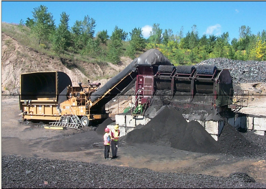
Ref: Krivit, D. (2007). Recycling Tear-Off Asphalt Shingles: Best Practices Guide . The Construction Materials Recycling Association
